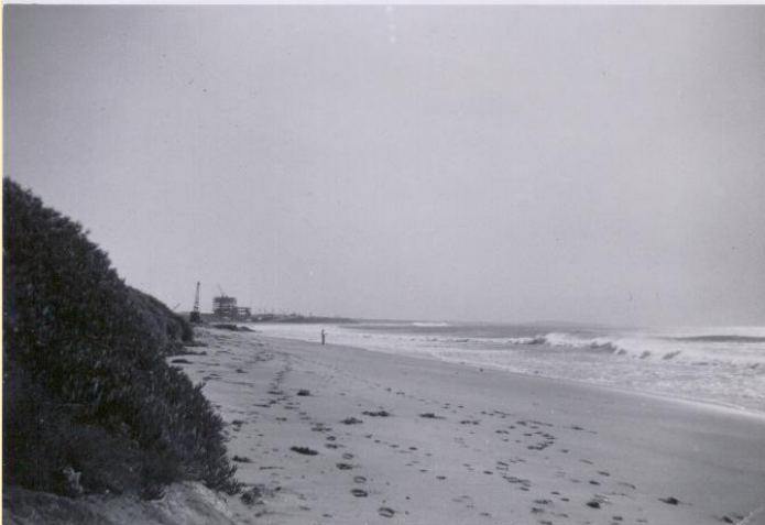
Carlsbad Power Plant being built
