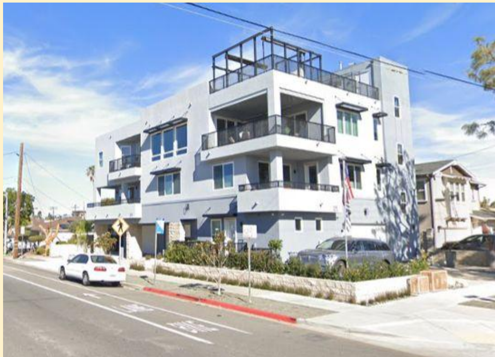
Apartment building on Harding and Pine Avenues
