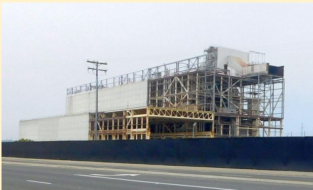
Remaining Encina Power Plant
