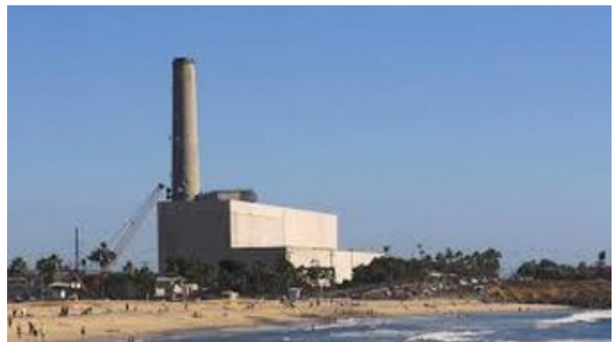
Carlsbad's Power Plant is 62 years old
