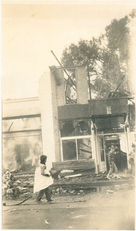
State Street Fire – 1927
