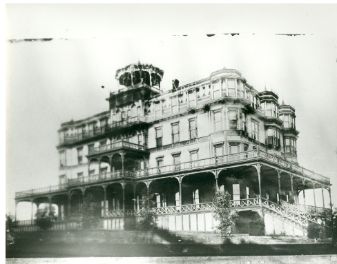
The Carlsbad Hotel, constructed in 1888, located on Grand and Highway 101, viewed looking northwest. This location would be directly across the street from present day St. Michael's Episcopal Church.
