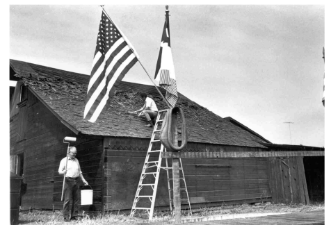
The Magee Barn getting a new roof
